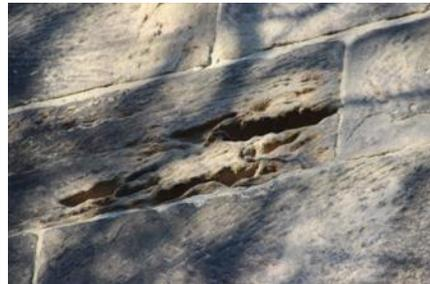
Stone jamb damaged in top corner to window SFW10.
