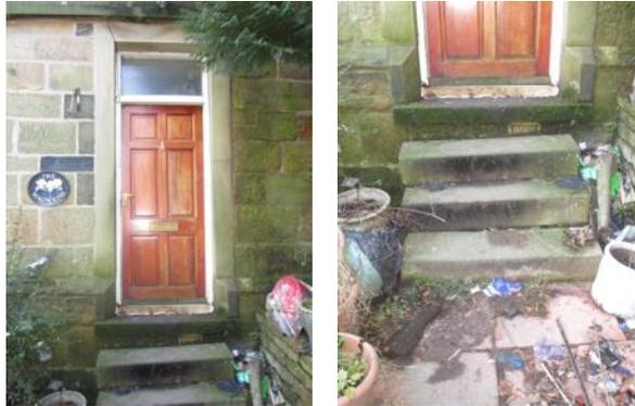
5.4 GFD4: Solid core timber single door. Paint finish is not good and missing in various places. Restricted access in this area didn't allow a close inspection but from a distance this door looks in fair condition.
