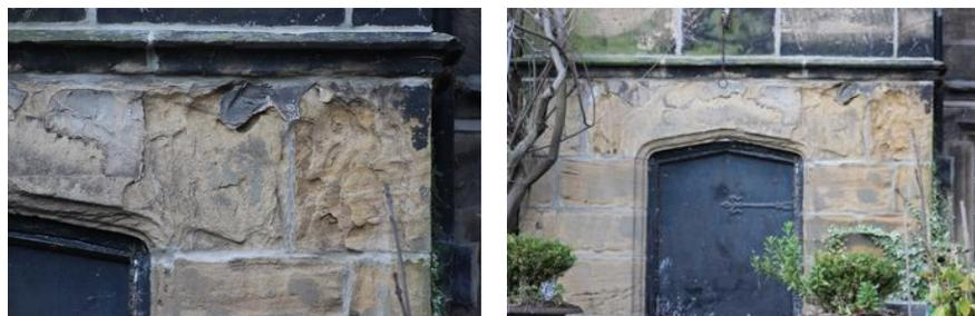
Iron lamp bracket is in poor condition and needs a full refurbishment. Lower string course over windows has wide cement rich pointing which is inappropriate and needs removing and repointing in a lime based mortar.
