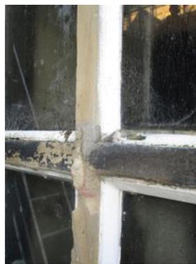
Window GFW5 Lower stone mullion and right hand stone transom are in poor condition, heavily eroded and unsightly with loss of definition and integrity. Replace stonework and refurbish windows
