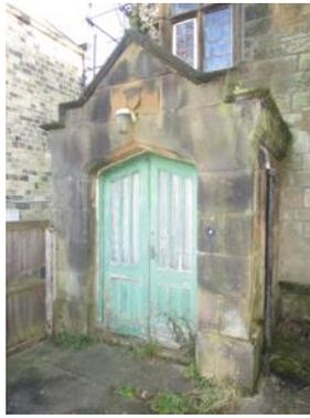
5.2 GFD2: Solid core timber double doors with glazed vision panels to each door. Paint finish is good. Doors look to have been recently installed. These doors are in good condition.
