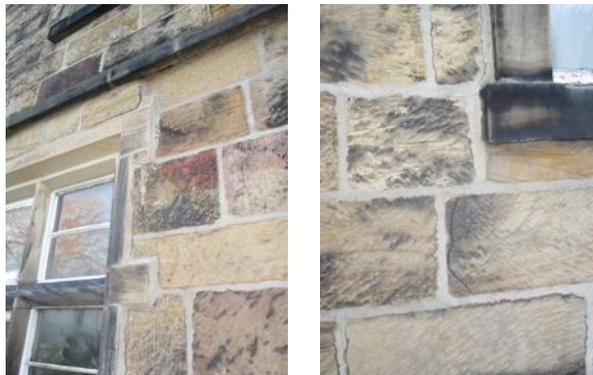
Light cracking within the vertical joint adjacent window FFW5 between stone jamb and facing stonework which ends just below cill level where there is a crack through 1 facing stone.
