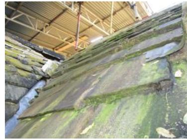
Roof B1: West side adjacent gable no. 3 area inspected from ladder and existing scaffold. The roof in this area is deteriorating badly and in very poor condition. Stone roof tiles removed in areas and covered with temporary sheeting. Both sides of the roof adjacent gable no. 3 are in poor condition with exposed rotten rafters and stone tiles missing, slipped and broken slate. Estimated that 40-30% salvageable where stone roof tiles are actually present for a reconstruction of the roofs.
