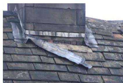
All the stone ridge sections appear to be present and mortar bedded. However, the ridge line does undulate due to poor workmanship as sections have been re-bedded, particularly adjacent the chimney on the South side. Also poor bedding and workmanship to the South end towards gable no. 1 and North end towards gable no. 2. Open pointing to the majority of joints.
