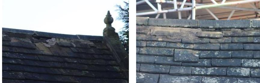
Stone water tabling to gable no. 2 west facing has open pointing with heavy mortar bedding and flaunching which has cracked and come away from the copings. On the east facing side there are less coping stones due to the abutment with the adjoining roof. Mortar bedding looks in poor condition and copings look loose. As the copings run down towards the adjoining roof the last coping is broken with some stone coping missing.
